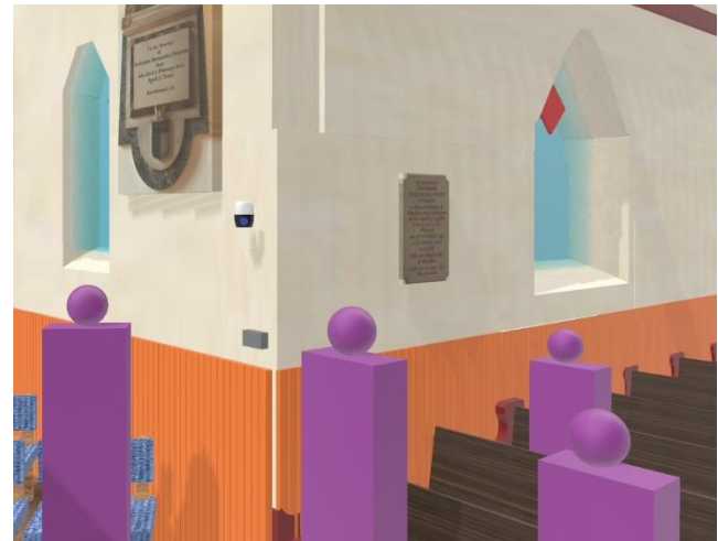
3 Impression of wall mounted PTZ camera in South Transept
