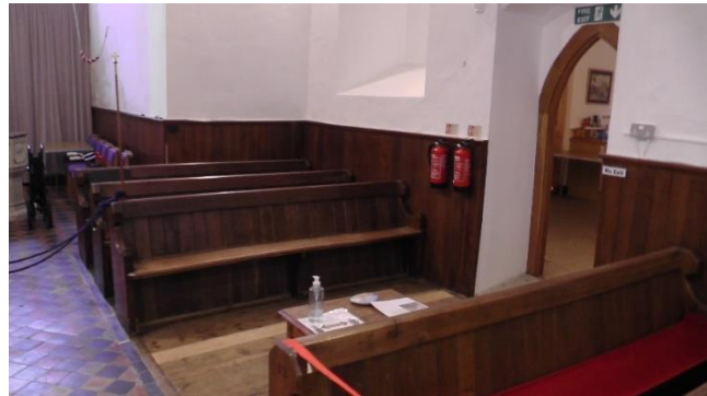
5 Existing (three) pews at proposed location of control area
