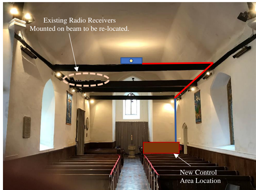
8 View of nave with proposed location of projector and new cable route.
